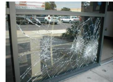
The window shown above was fitted with security tint which prevented the glass from shattering.
