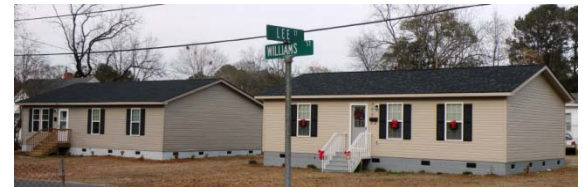
New CDBG homes constructed on Williams Street
