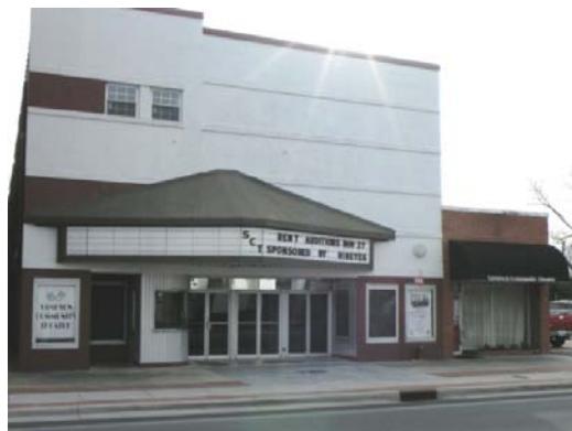
Sampson Community Theater, 115 Fayetteville Street
