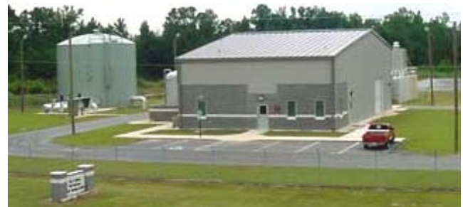
Well Field East Water Production Plant on Clive Jacobs Rd.
