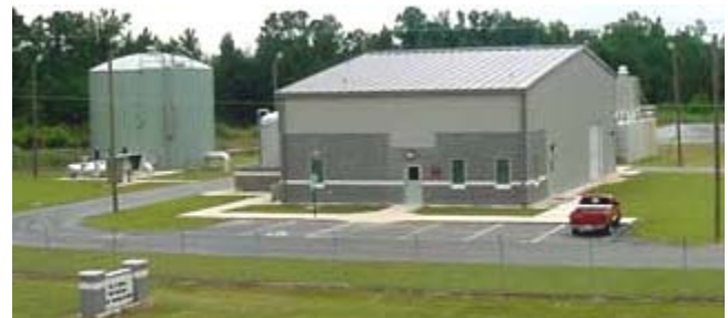
Well Field East Water Production Plant on Clive Jacobs Rd.
